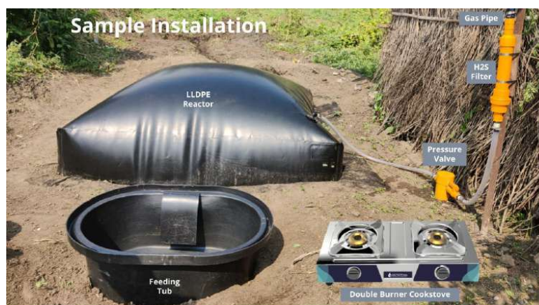
Figure 7. On-field installation of a Flexi biodigester system
